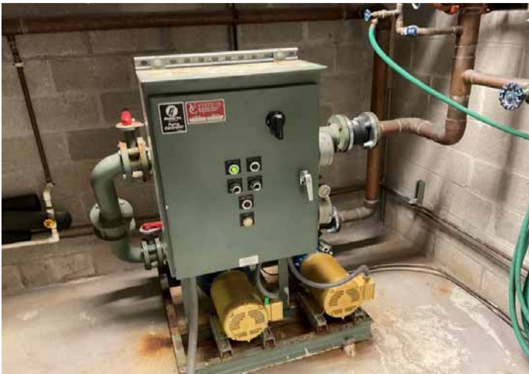
Domestic Water Booster Pump System
