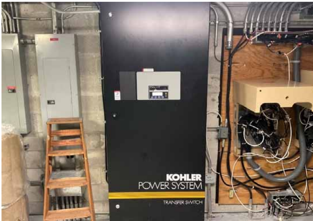
Generator Transfer Switch
