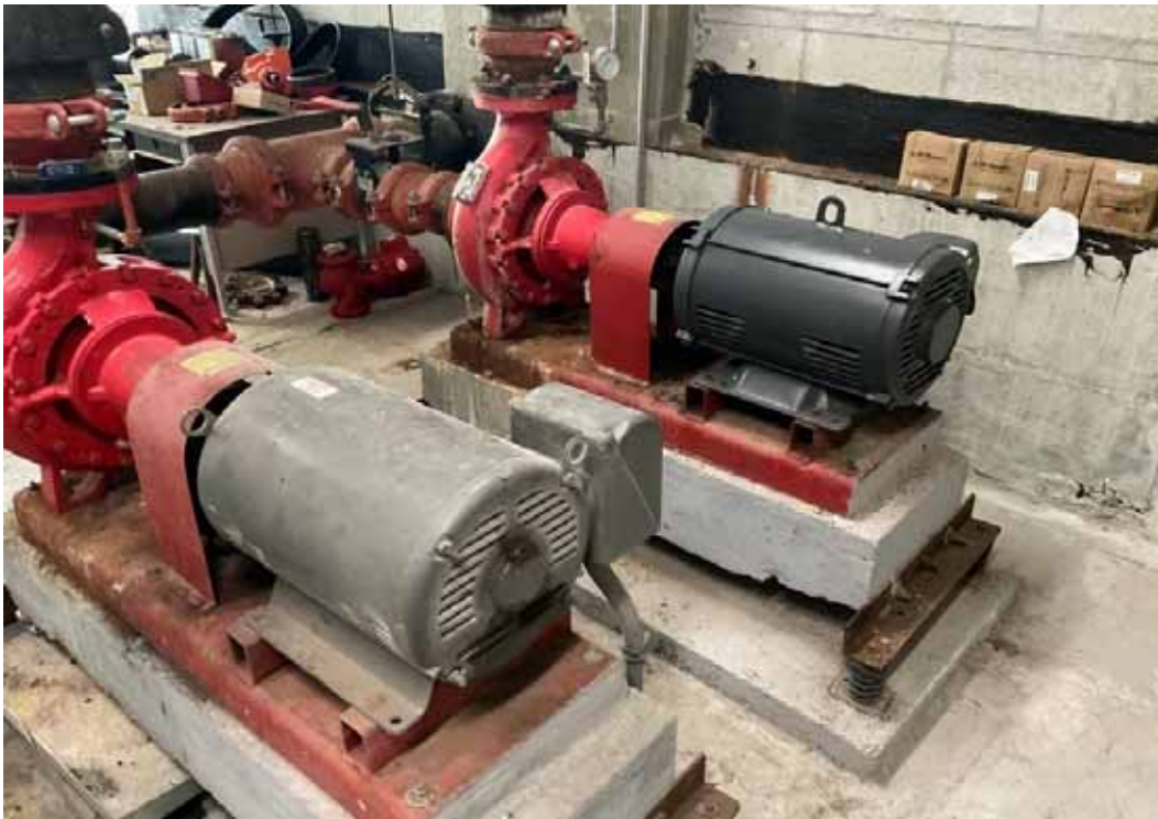
A/C Condensing Pumps
