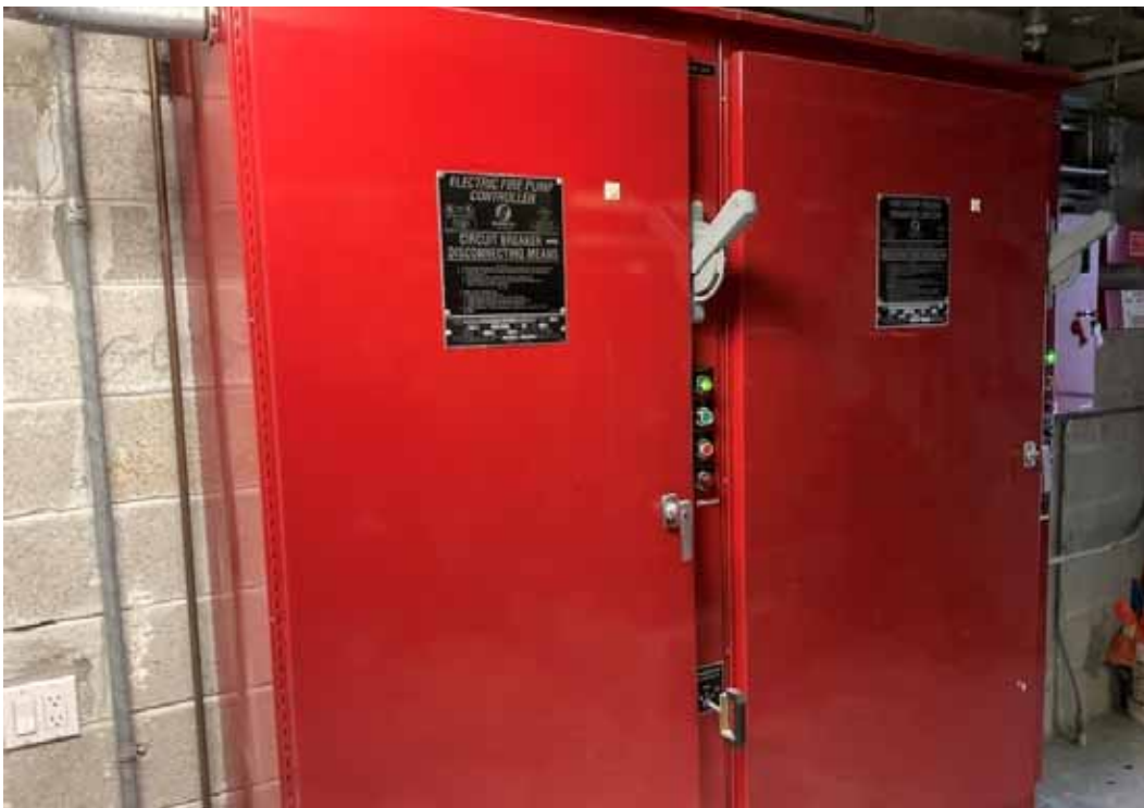
Fire Pump Controller
