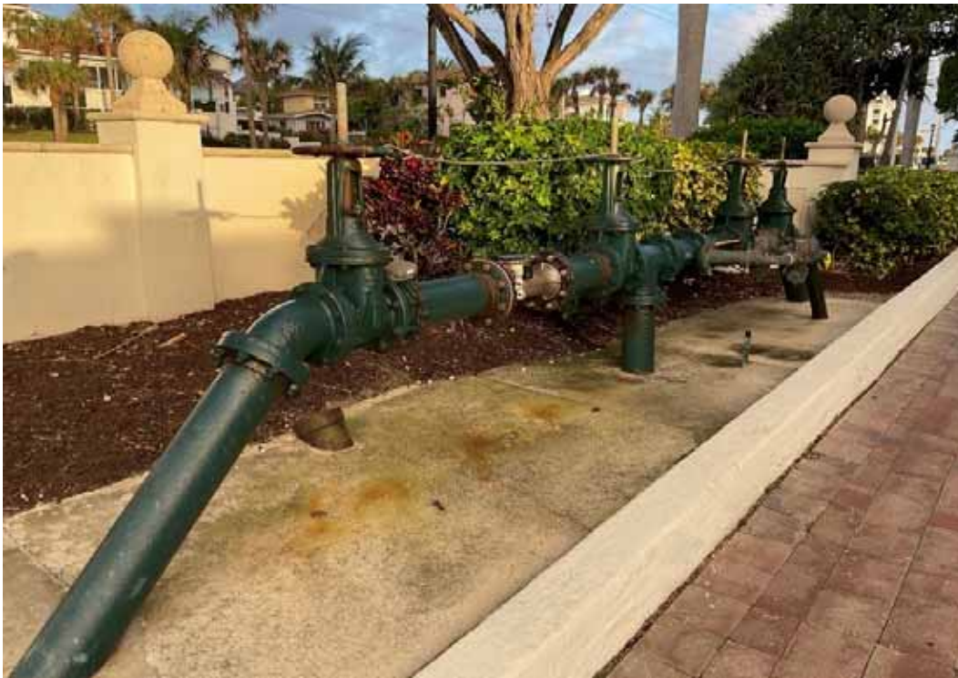
Backflow Preventer - Fire & Dom Water
