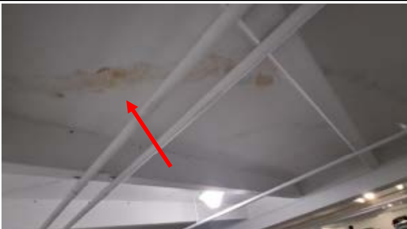
Water Stains at Overhead Concrete Slab, Parking Spot #80
