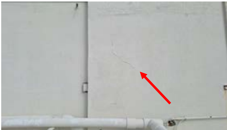
Stucco Cracks at Exterior Wall at Roof Elevator Room
