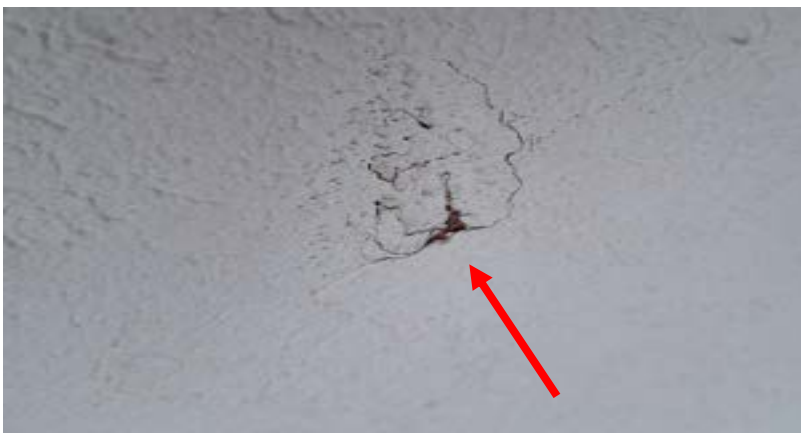
Stucco Cracked and Missing at Balcony Wall
