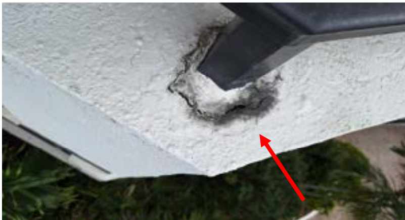
Deteriorated Rail Post Pocket at Balcony with Water Intrusion
