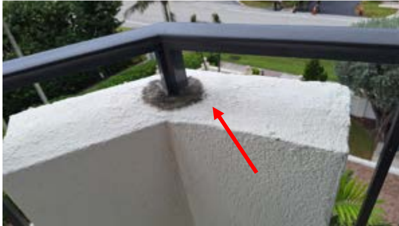
Deteriorated Rail Post Pocket at Balcony with Water Intrusion
