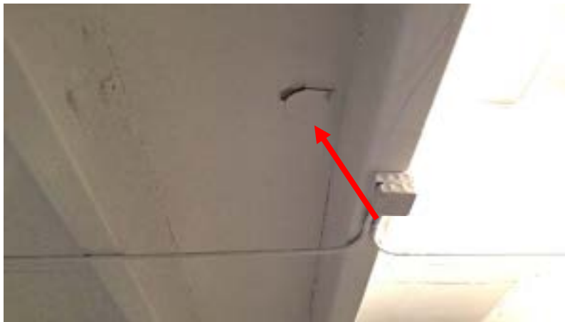
Overhead Concrete Slab Spall, Parking Spot #85
