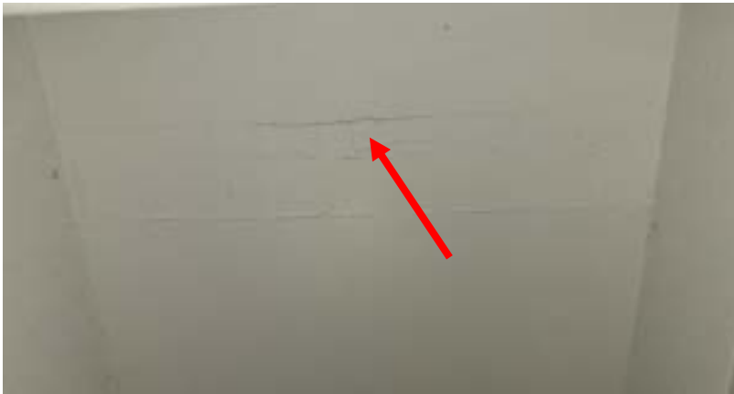
Cracks In Overhead Concrete Slab, Parking Spot #49
